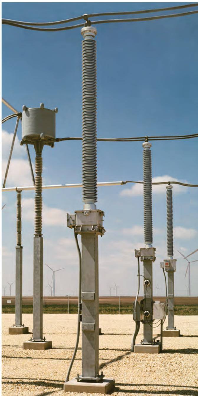
**Trench is the recognized world leader in the design and manufacture of Capacitor Voltage Transformers (CVT's) and Coupling Capacitors (CC's). Trench has been manufacturing CVT's since the early 1970's and installations in virtually every country in the world attest to their acceptance and reliability. In order to maintain and enhance technical excellence while retaining commercial competitiveness, product refinements must be ongoing.**
